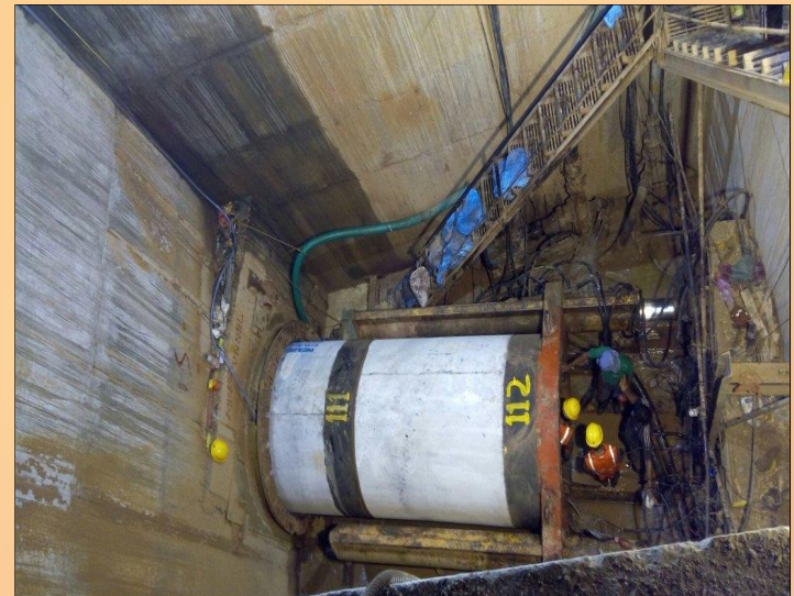
VMSS – Micro Tunneling Vadodara
