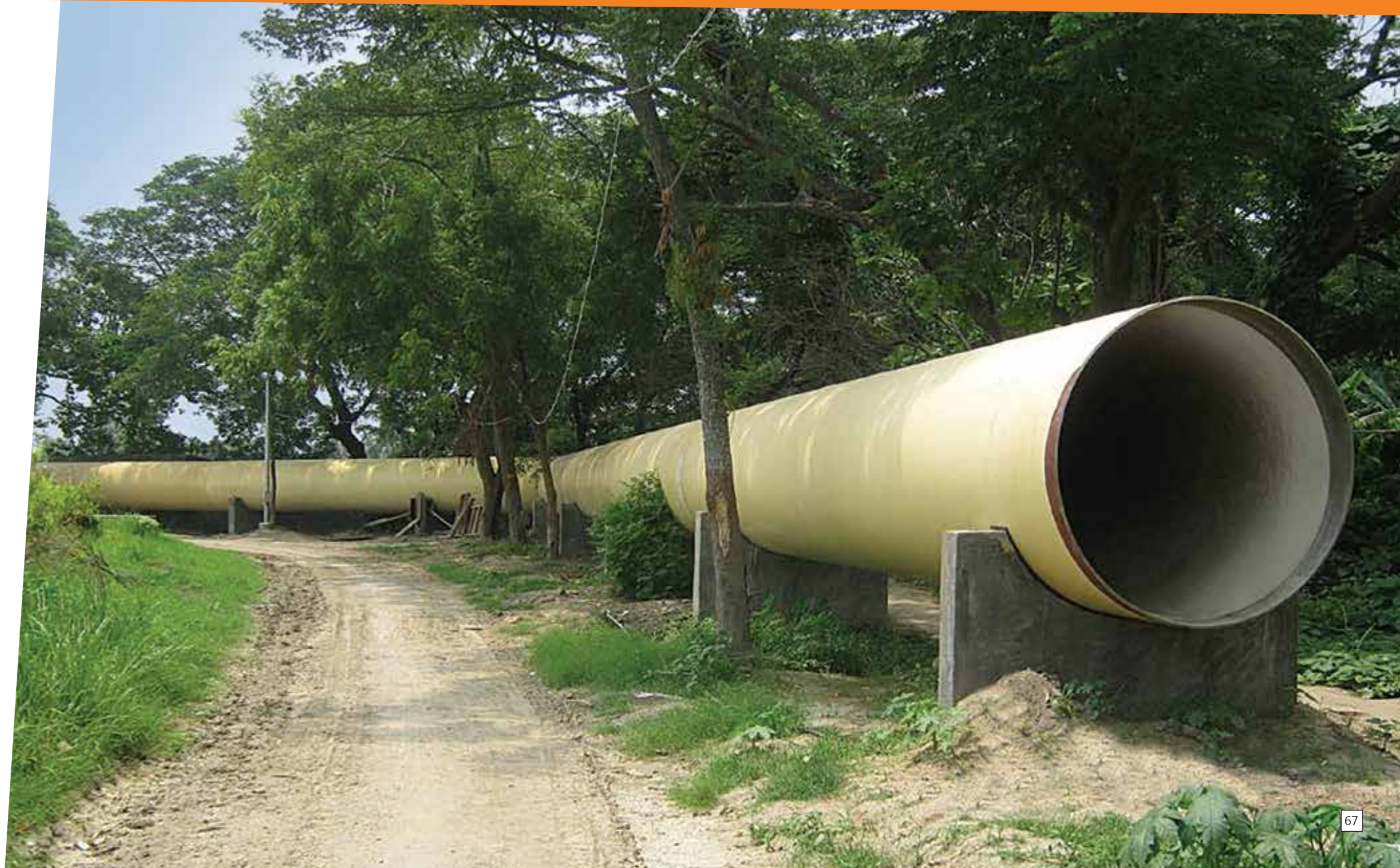
Laying of Tallah Palta Dedicated Water Transmission Main for KMC
