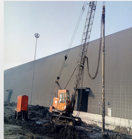
Stone Column Work at Jindal Steel
