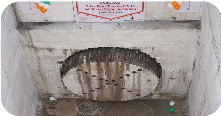
MCGM micro tunnel breakthrough in Mumbai
