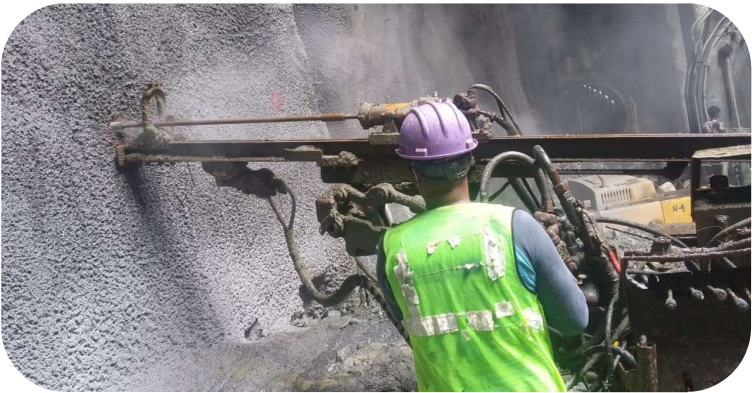
Rock bolt drilling in Mumbai UG station
