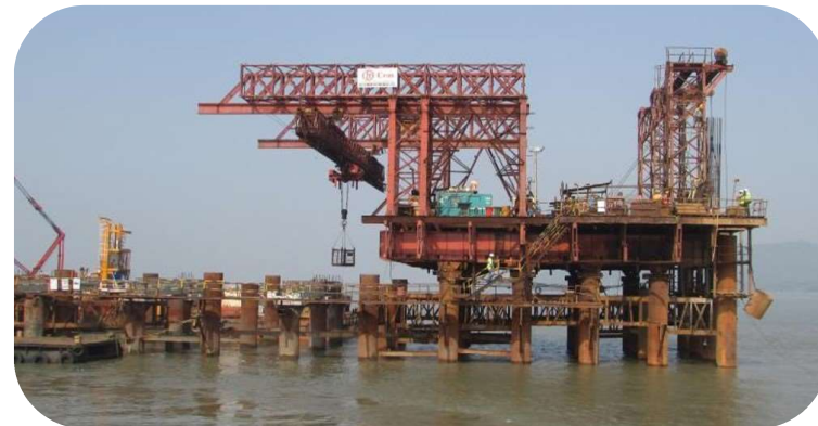
JNPT, Liquid Jetty in Mumbai, Maharashtra
