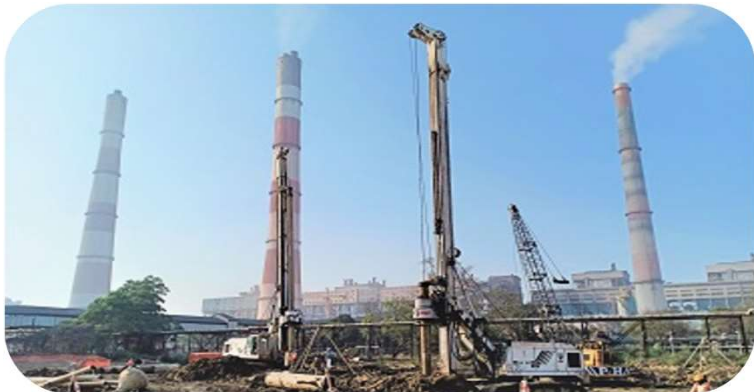
Unchahar project in Uttar Pradesh
