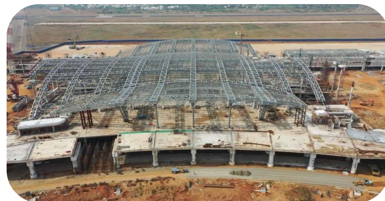
Trichy airport project in Tamil Nadu
