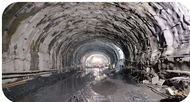
Sivok Rangpo railway tunnel project
