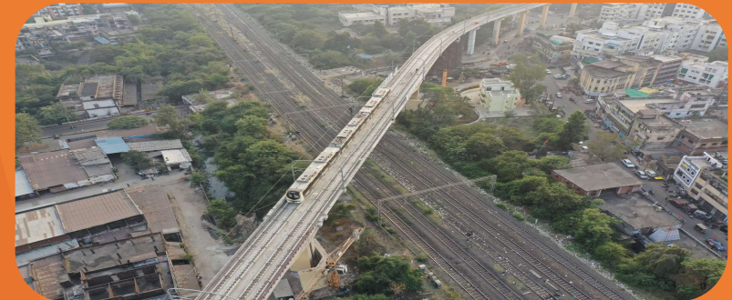
Nagpur Maha Metro cantilever bridge in Maharashtra
