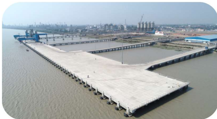
Haldia Multi Modal IWT terminal in West Bengal
