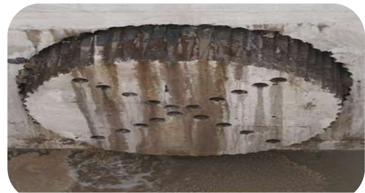
MCGM micro tunnel breakthrough in Mumbai
