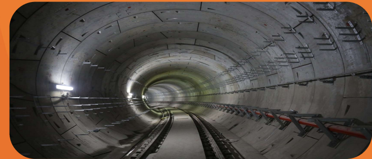
Mumbai Metro Underground tunnel in Maharashtra
