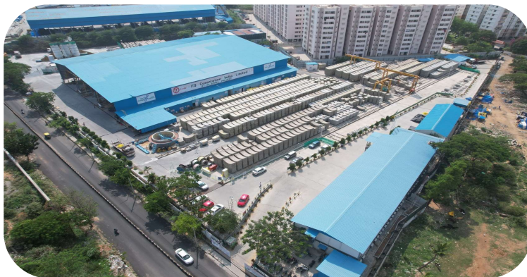
Bengaluru underground metro casting yard
