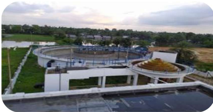
Water treatment project in Agartala, Tripura
