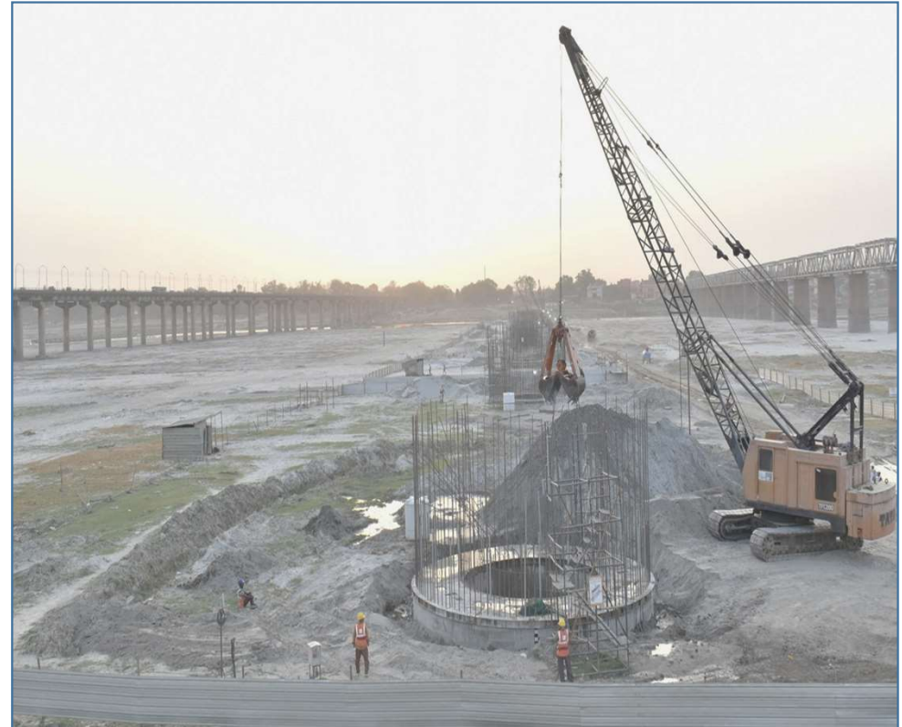
Ganga Steel Bridge project in Uttar Pradesh
