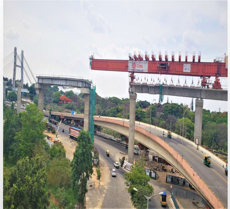
LG Crossing Over Existing Flyover, BMRCL Project
