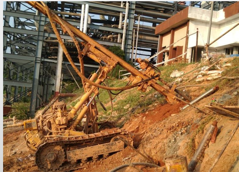
Drilling for Slope Stability at MRPL, Mangalore
