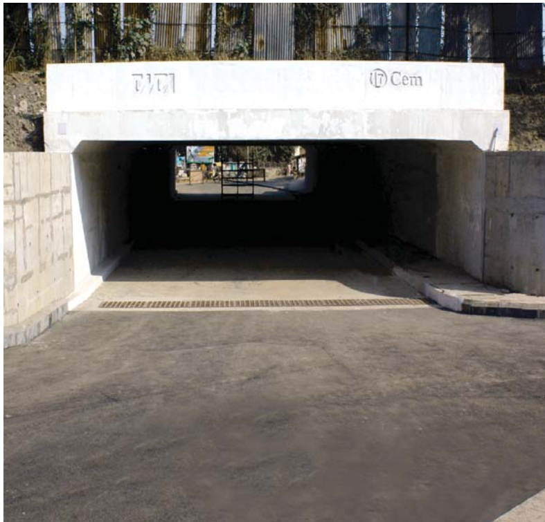
Box Pushing below Rail Track, Kolkata
