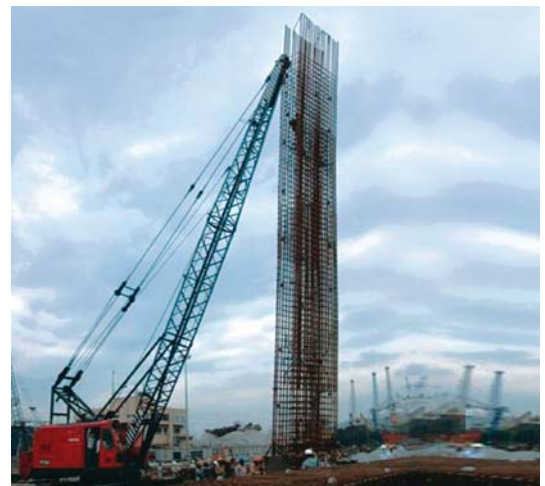
Construction of Diaphragm wall, Delhi
