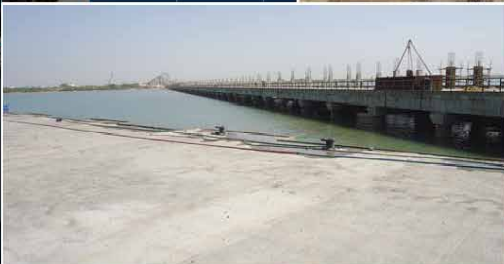
Jetty for Jaypee Cement at Gujarat
