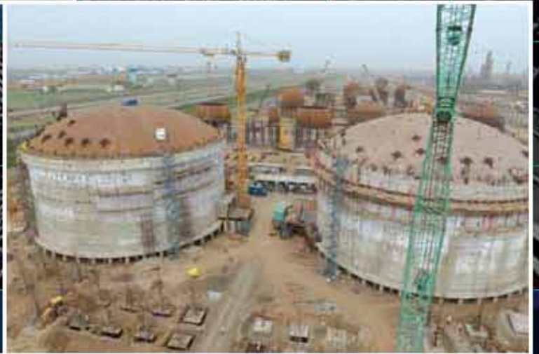
Double Walled Pre-stressed Cryogenic Tank at Dahej, Gujarat
