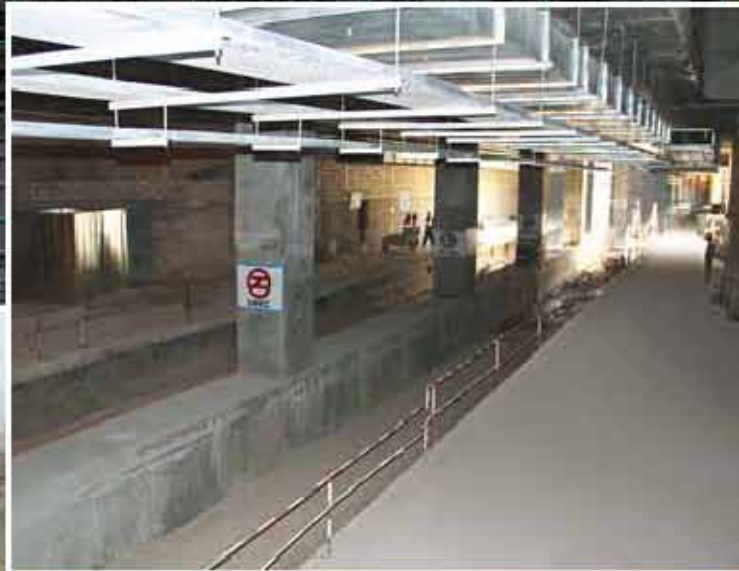
Inside view of Jaipur Metro Station, Jaipur, Rajasthan
